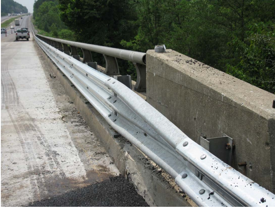
Figure 3.2-Bridge rail retrofit with thrie beam
